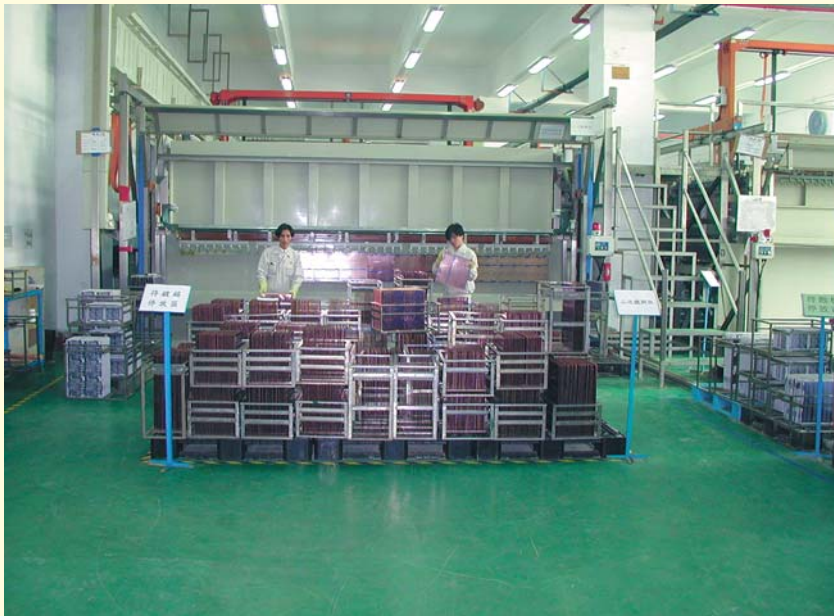
Plating tanks as big as your living room in the newly installed High Capacity Plating plant!
